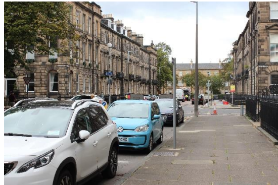
Figure 18 Manor Place, east side, looking north.
