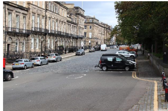
Figure 33 St Colme Street, south side, looking east
