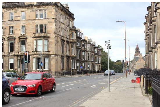
Figure 13 Palmerston Place, east side, looking north.
