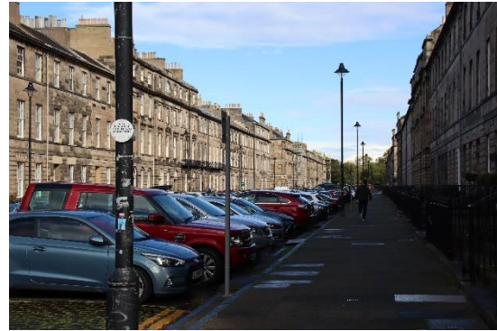
Figure 61 Great King Street, south side, looking east
