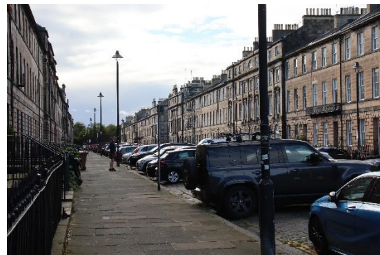
Figure 63 Great King Street, south side, looking west
