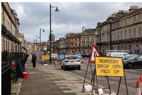
Figure 20 Melville Street, north side, looking east
