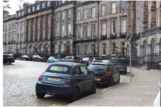
Figure 31 Moray Place, north side, looking west.
