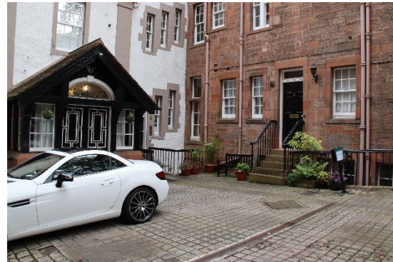
Figure 81 Ramsay Gardens, looking north-east
