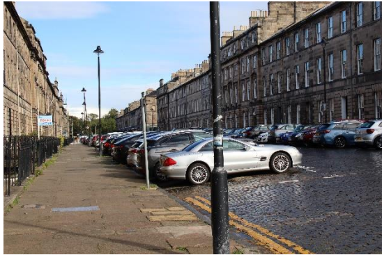
Figure 60 Great King Street, north side, looking east
