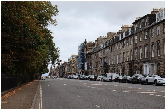
Figure 48 Queen Street, north side, looking east
