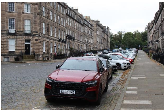
Figure 50 India Street, east side, looking south
