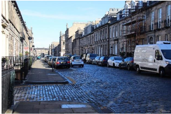
Figure 64 Northumberland Street, north side, looking east
